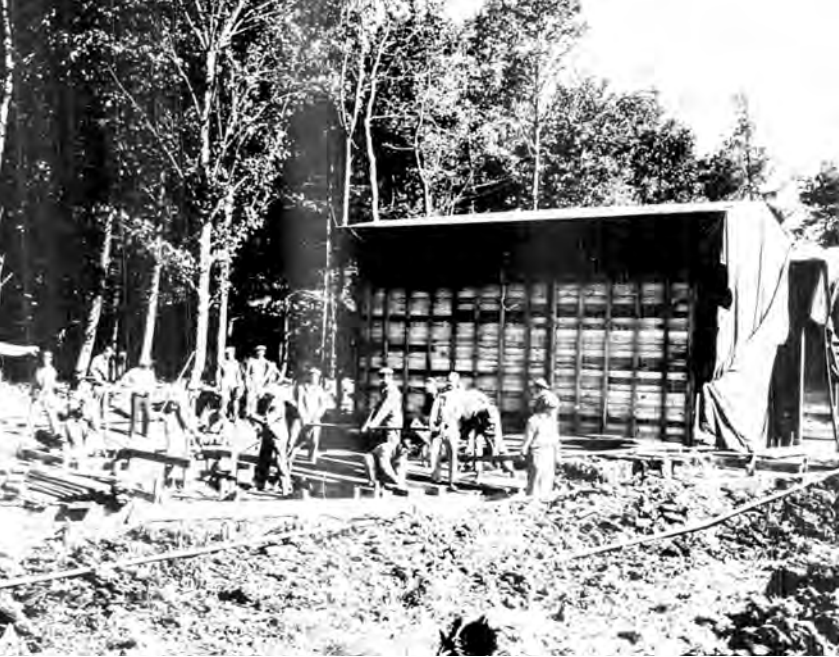
Facility Construction Langford Lodge, Lockheed Overseas Corporation Annual Report 1942-1943. 1943, National Archives
